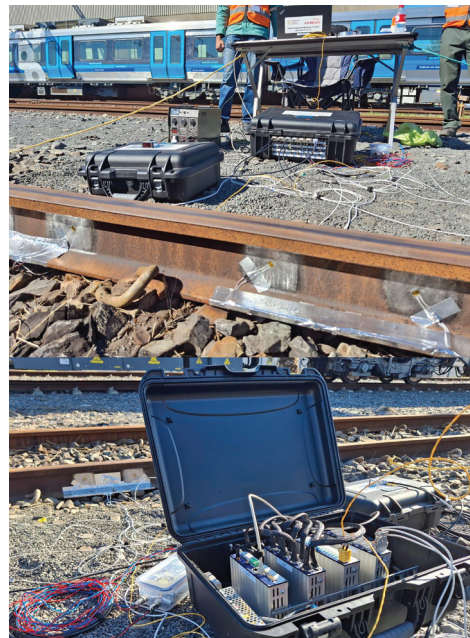
Figure 46: Newly acquired equipment put to use on site.
